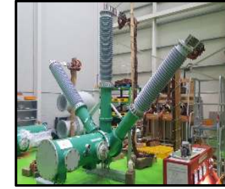
[Temperature rising test]
