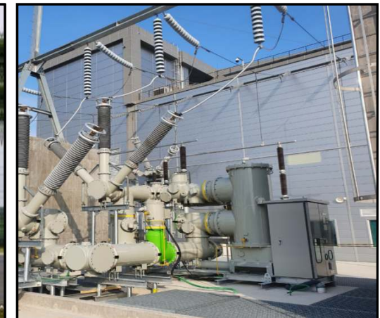
[Installation of ECO 170kV GIS]
