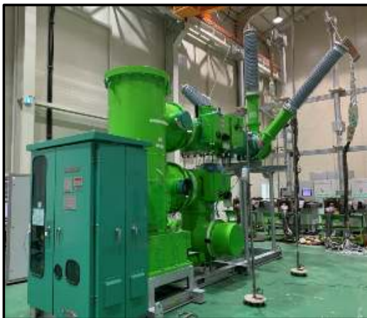
[GIS Temperature-rise test]
