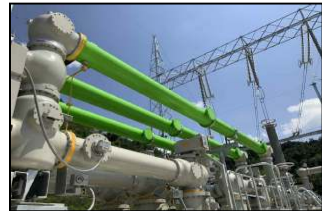
[Development and installation of the pilot project of 362kV 63kA 6300A GIB, Jun 2019~]
