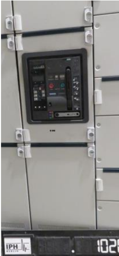
Circuit-breaker section
