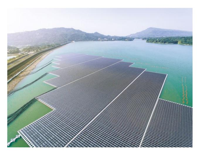
An electricity company asked CESI to create guidelines for assessing the potential for installing floating solar photovoltaic (PV) installations on hydroelectric reservoirs from sustainability, technical and economic perspectives.
